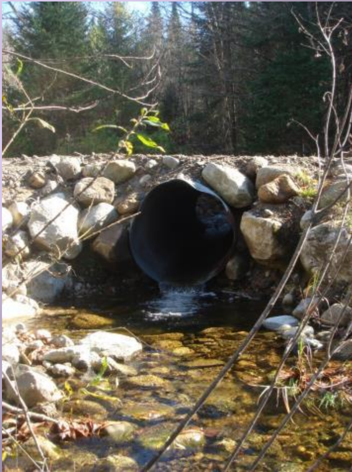
Pre-replacement – looking upstream October
