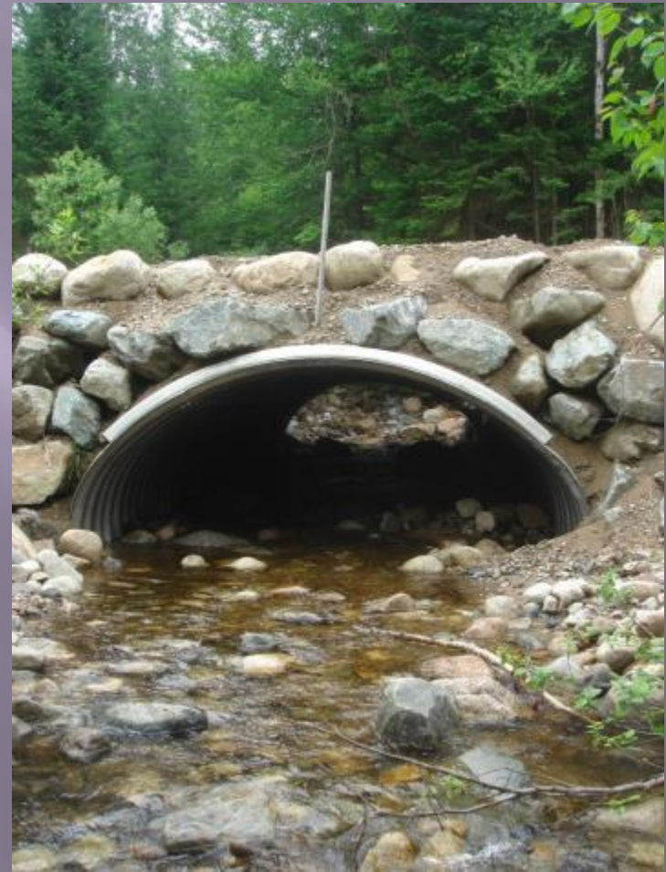
Post-replacement – looking upstream July 2013
