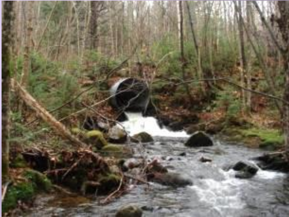
Pre-removal – looking upstream
